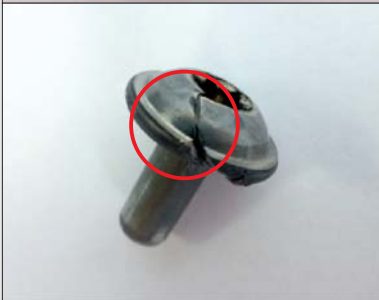
Typical cracked parts that were detected
